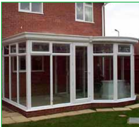
Flexi roof & Colwall combined
