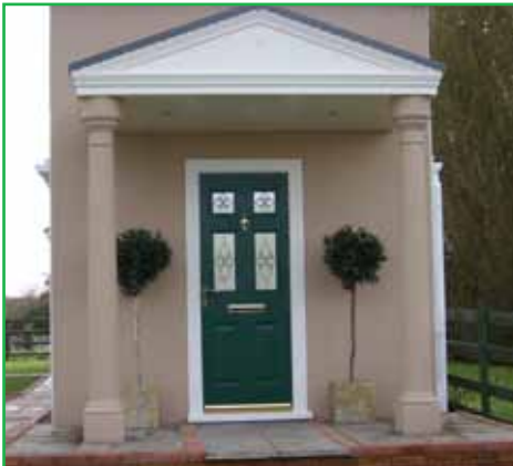
Alderbury & Smooth columns painted
