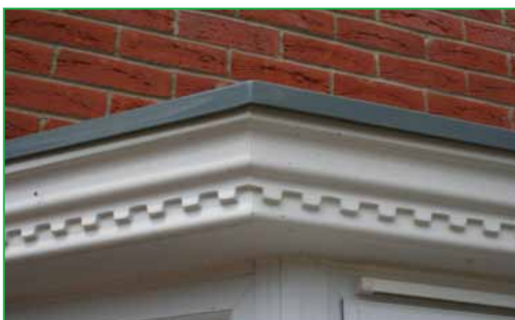
Victorian fascia close up
