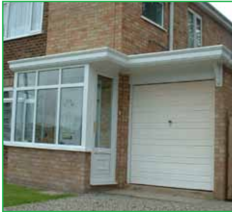
Flexi porch extended fascia over garage
